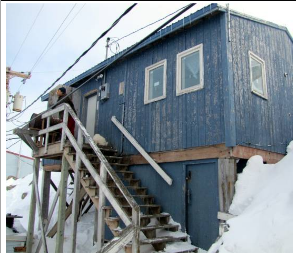
Diomedede's IRA Office Building
