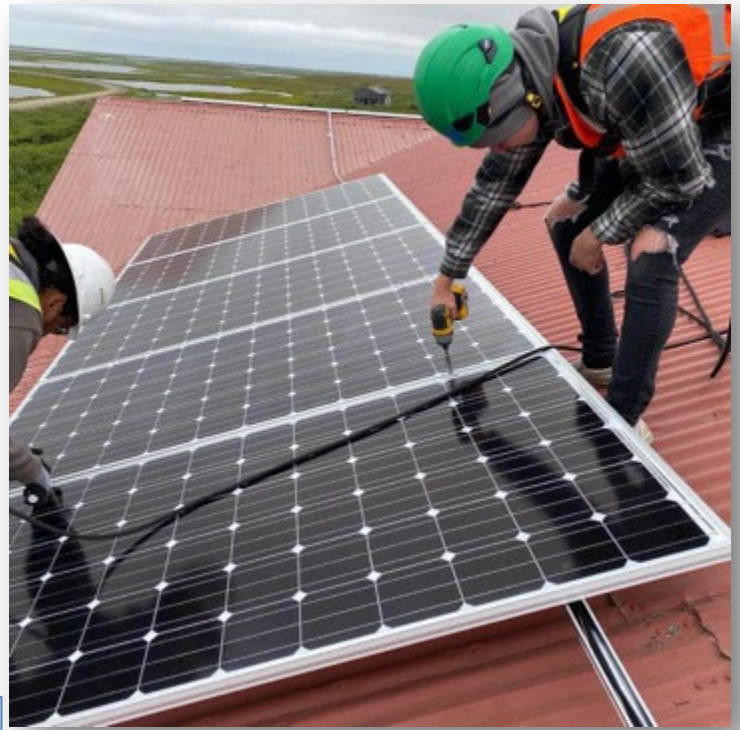
(Brewster Bohn assisting the rooftop solar panel install July 2021)
