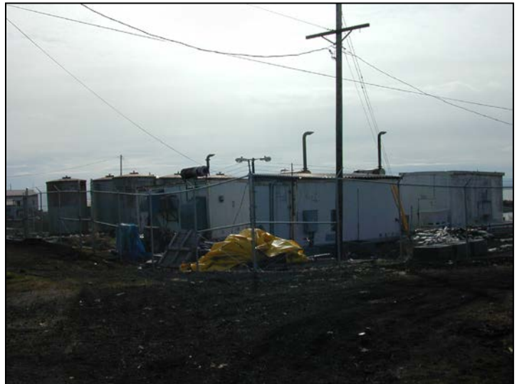
Decommissioned AVEC power plant. Power is now provided by the Stebbins power plant through an intertie.
