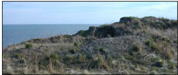
The ground southeast of St. Michael has eroded and sunken over the last few years.
