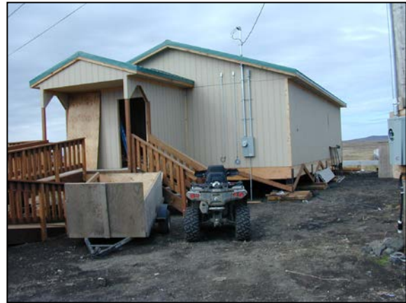
BSRHA house in progress for Martin P. Andrews, Sr.
