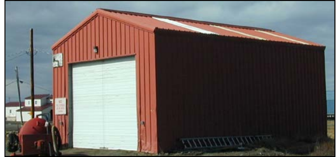
The old airport building now serves as the City of St. Michael equipment storage facility.
