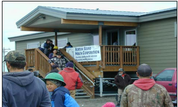
New Norton Sound Health Corporation Triplex in St. Michael, AK and the first paraprofessional housing in the Bering Straits Region.
