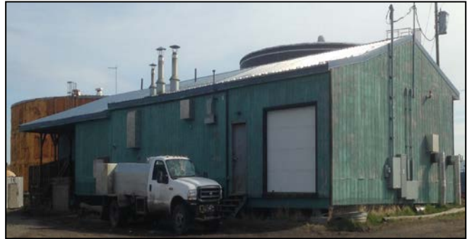
Water Tank building and office and includes the laundromat.
