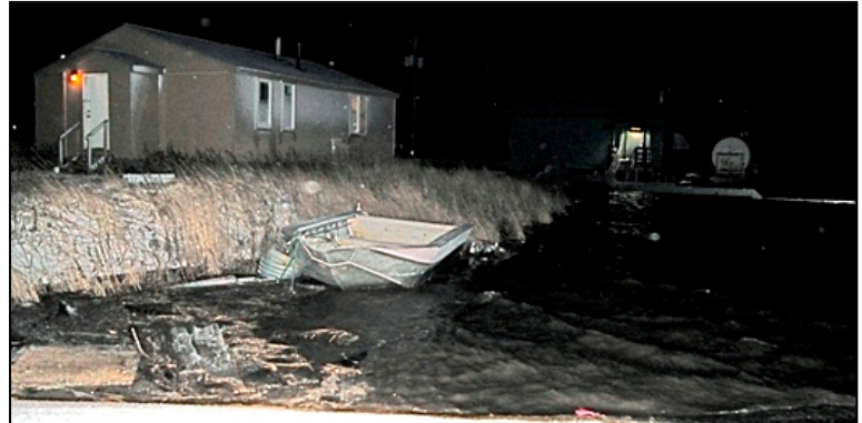
Fred Oyoumick's residence with the St. Michael sewage treatment plant and water and sewer utilidors near Sidewalk Street, all areas near extensive shore erosion.
