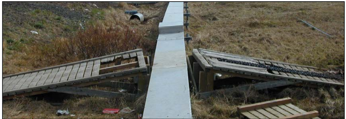
The above ground vacuum sewer system poses challenges for navigation and board walks and ramps need regular maintenance to insure safety.
