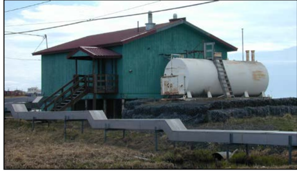
The St. Michael City Water Pump House for the vacuum flush sewer system.
