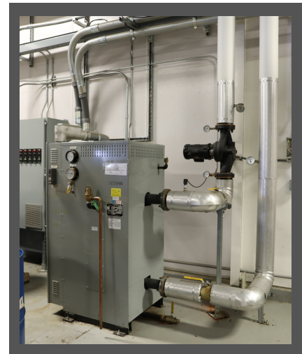
HEAT RECOVERED - This unit collects heat from the diesel generators in Unalakleet and distributes that heat to facilities around the community. Photo by Kawerak, Inc.
