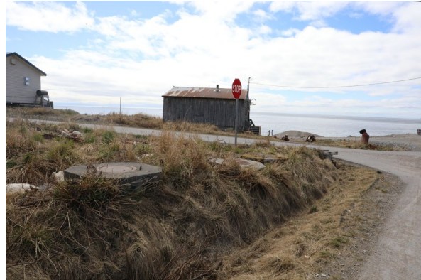
Figure 13 Sewer manholes are shown elevated from the eroding ground.
