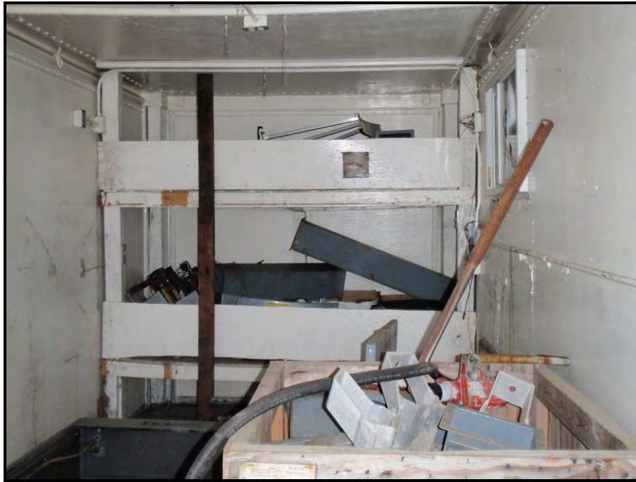
Photograph 13: Equipment inside the CONEX building.
