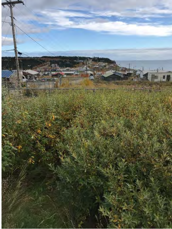
Photo 1: Overhead view of tank farm from west looking east
