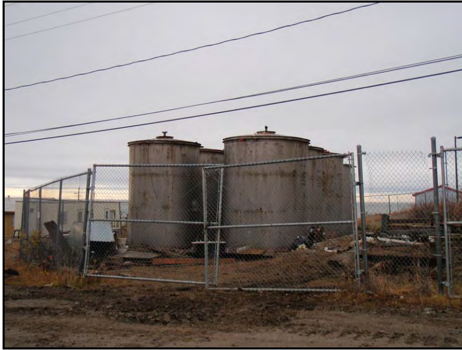
Photograph 1: Vertical ASTs on the east side of the property (photograph taken looking south).
