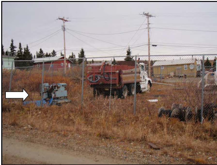
Photograph 5: An old generator was present on the site. No stained soil was observed next to this generator.
