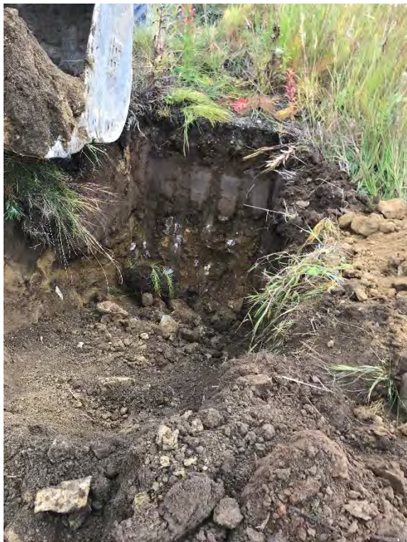
Photo 7: Test pit 1 – typical presentation
